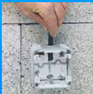
2/ Insert the cable through the end cap
