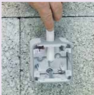
2/ Insert the tube through the end cap
