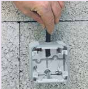
2/ Insert the cable through the end cap
