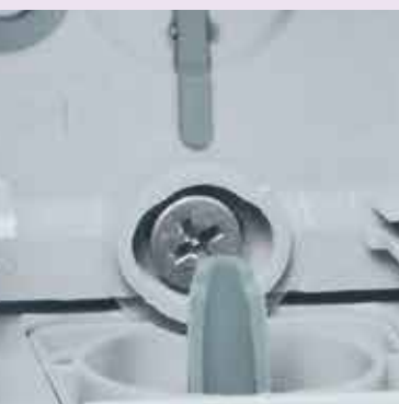
Visible and accessible fixing points; identical to the Plexo 55
