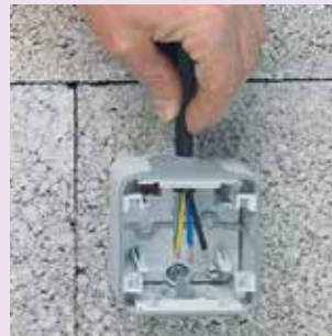
3/ The membrane of the end cap ensures IP 55 protection of the installation
