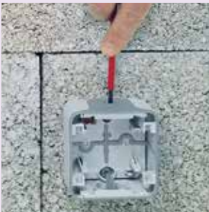
1/ Pierce the end cap using a screwdriver
