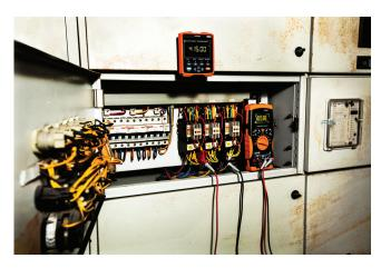
Figure 3. Monitoring handheld meter readings via the U1115A remote logging display
