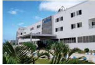
Rudrapur Plant (Green Building)
