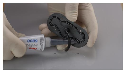
Figure 7: 3M 5200 Marine Adhesive Sealant provides the strength required to bond through-hull fittings and reliably seal below-waterline applications over the long term.
