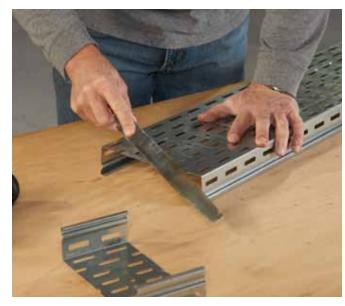
CUTTING STRAIGHT SECTIONS FOR ELEVATION CHANGES
