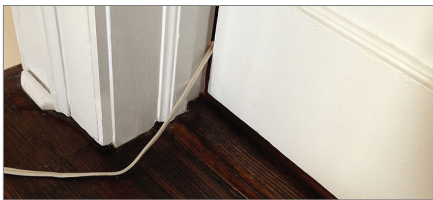
At loose electrical connections or cords damaged by doors closing on them
