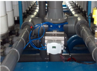
Designed for controlling process valves such as a butterfly valve across a wide range of industry sectors
