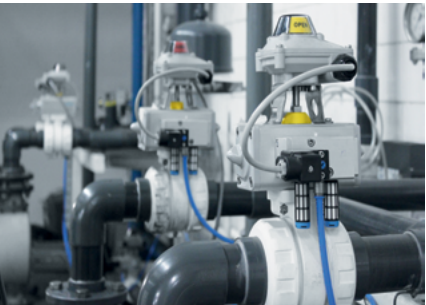
Actuated polymer valves for chemical applications
