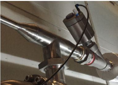
Shut-off control for glycol used in food productionh
