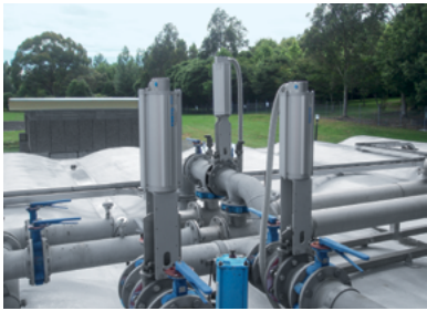
Controlled sluice gate for flowrate of return sludge at a wastewater treatment plant
